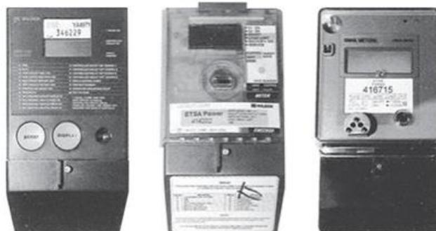
If you have an electric hot water or solar system, you may need to press a button to display the electricity meter read and continue to press it through a few screens until the reads for each register are displayed.
